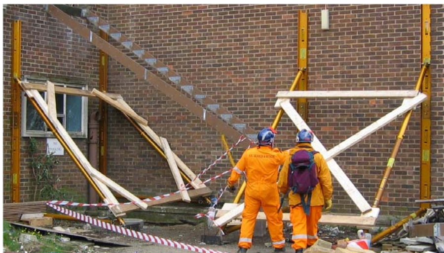
Figure 1: [SOP_SHO002] Raker Shoring in place
