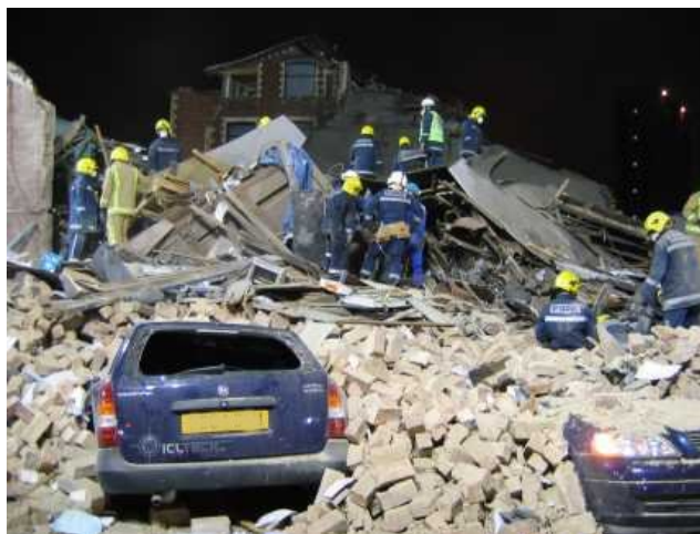
Fig 1: Early Stages of a Collapse Operation
